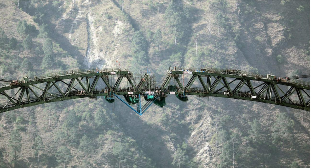
Construction of Chenab bridge has lasted nearly two decades. With the arch in place, its chords are now due to be filled with concrete to improve wind stability.
