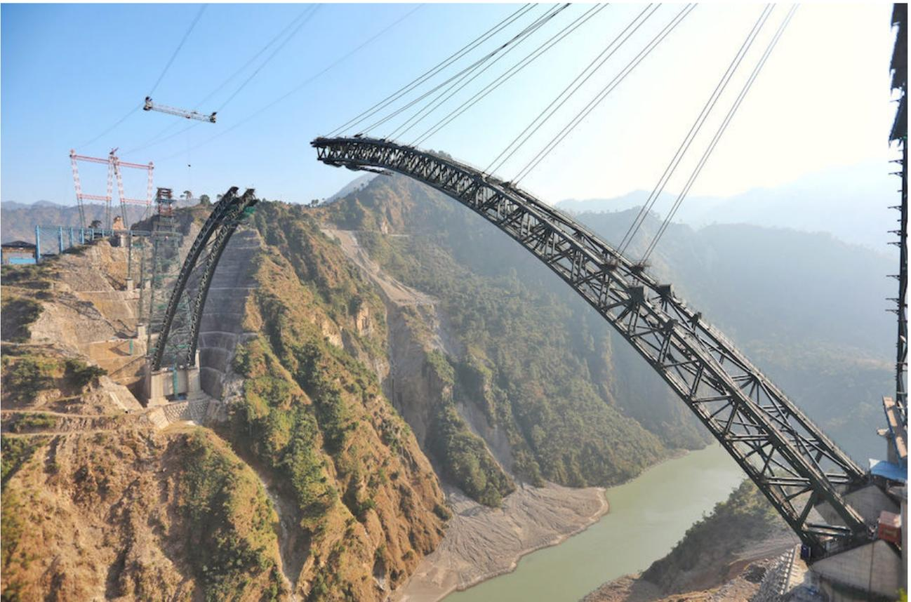
Bridge will be part of 272-m railway connecting Kashmir to Indian network. Arch sections traveled to their final positions along four cables strung between all steelwork towers about 130 m tall.
