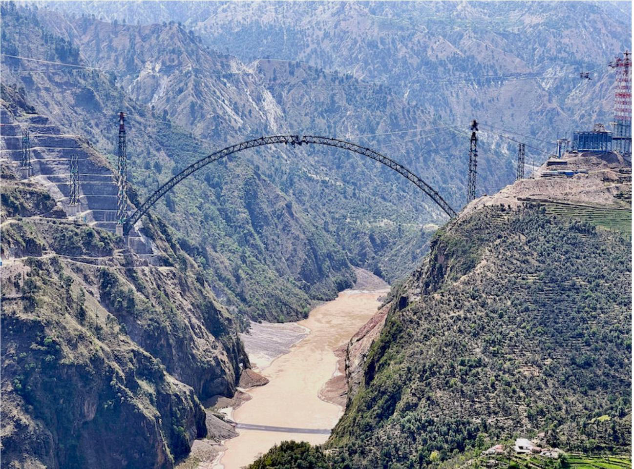
Arch bridge rises 359 m above valley floor. More than a million tonnes of earthmoving and countless rock bolts were needed to cut and stabilize steps in the slopes.
